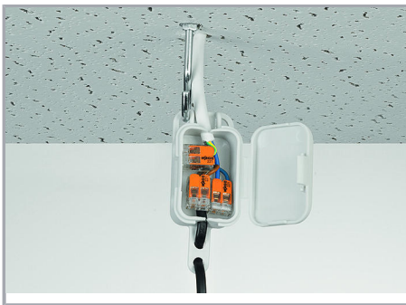
Pendant light connection in a suspended ceiling
